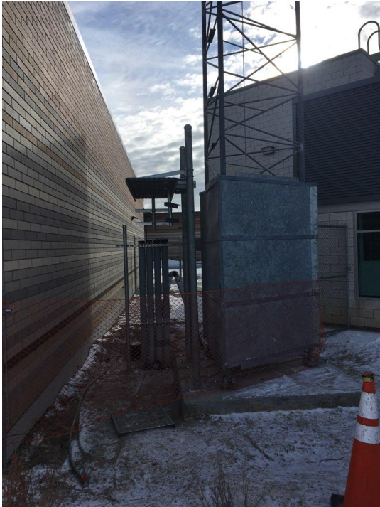
Figure 4 - Conduit and ice bridge construction at the base of the tower
