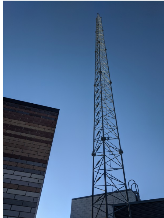
Figure 5 - Newly stacked tower at the Justice Center
