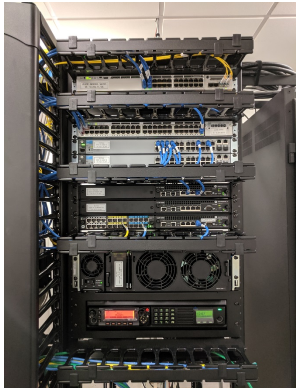
Figure 1 - Network and radio console equipment
